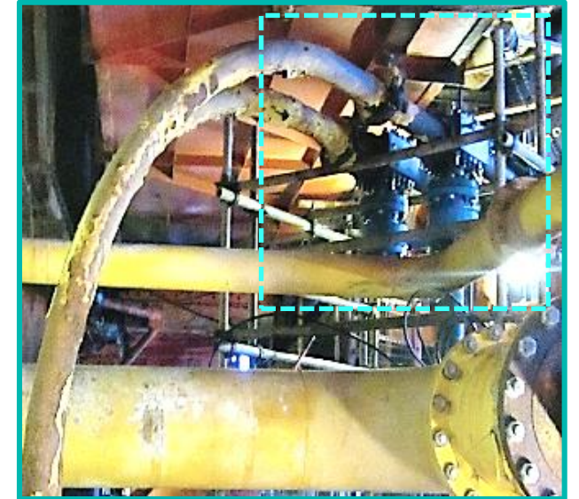
Flowlines with mechanical tie-in clamps and BISEPs installed
