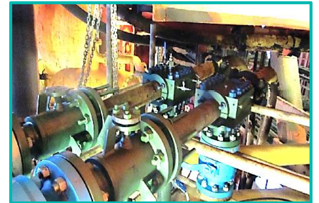
Flowlines isolated, mechanical connectors & valves installed
