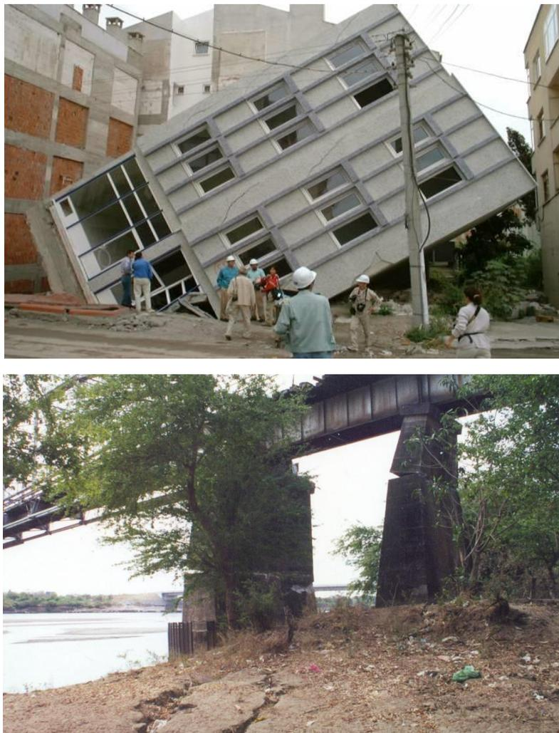
Figure 3. Effects of soil liquefaction. *Upper:* A building sunk into liquefied ground; *Lower:* Liquefaction-induced lateral spreading causing damage to bridge piers.
