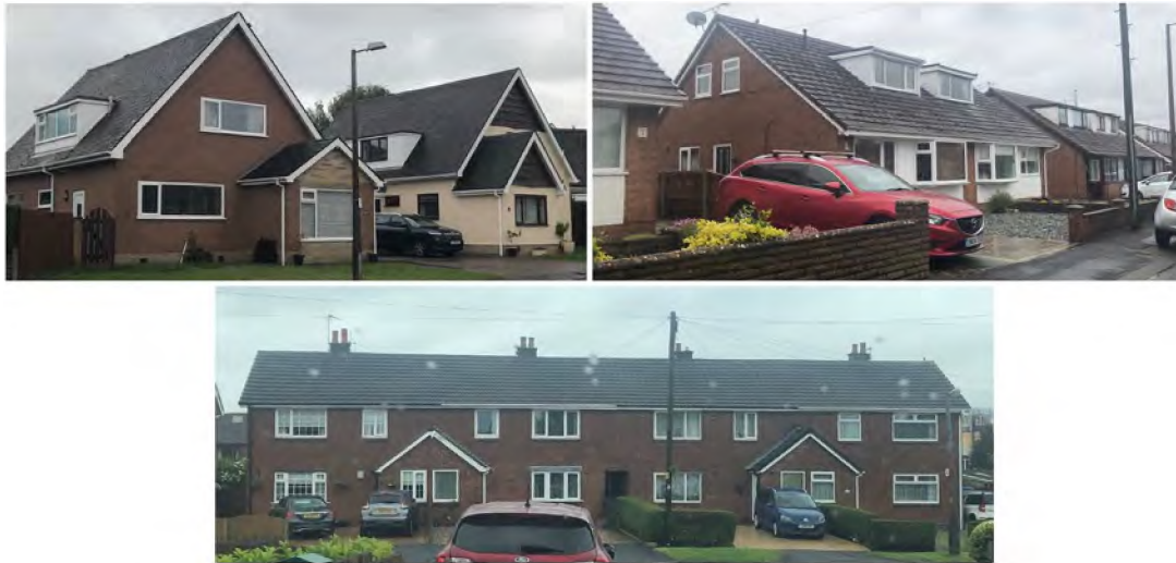
Figure 5.14. Modern masonry housing (terraced, semi-detached) without tall brick chimneys.
